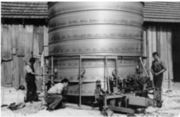
Fig. 9. Spiral -fold silos: Xaver Lipp's first spiral-fold silo, 1969 [49].
